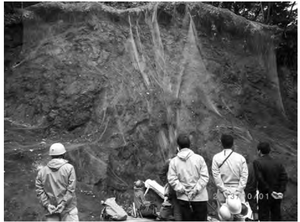
図 39 北海道胆振総合振興局の視察 (2013.10.1) Fig.39 Inspection by the Hokkaido government Iburi General Subprefectural Bureau (Oct. 11, 2013).
